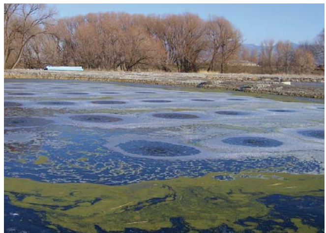
Fully submerged Bio-Domes in Wellsville, Utah.
