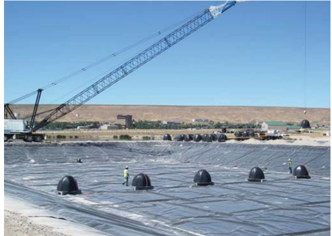
Bio-Domes are installed with a crane at Jackpot, Nev.
