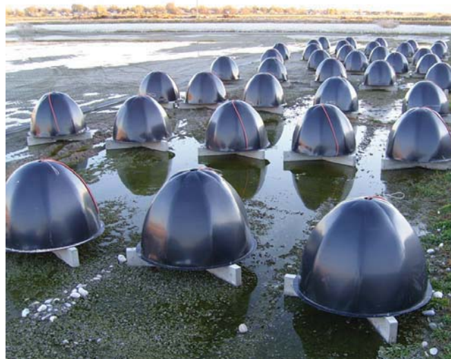
Pollution-eating, igloo-shaped devices nicknamed Poo-Gloos sit in an unfilled sewage lagoon in Plain City, Utah, before the lagoon is filled. (Photos and illustration courtesy of Waste Compliance Systems, Inc.)
